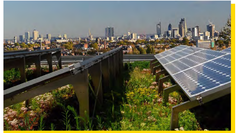
Combined green roof with photovoltaic panels
